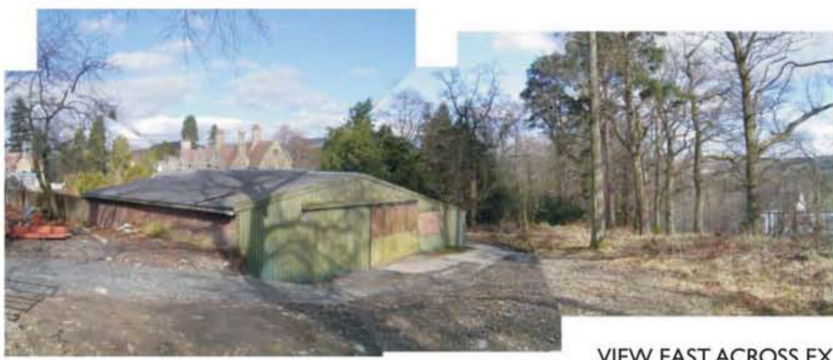
VIEW EAST ACROSS EXISTING SHED
